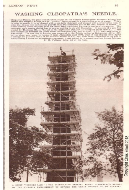
A GIANT "NEEDLE-CASE" THE SCARFOLDING ERRECTED ROUND CLEOPATRA'S NEEDLE ON THE VICTORIA EMBANKMENT TO ENABLE THE GREAT OBELISK TO BE CLEANED.
